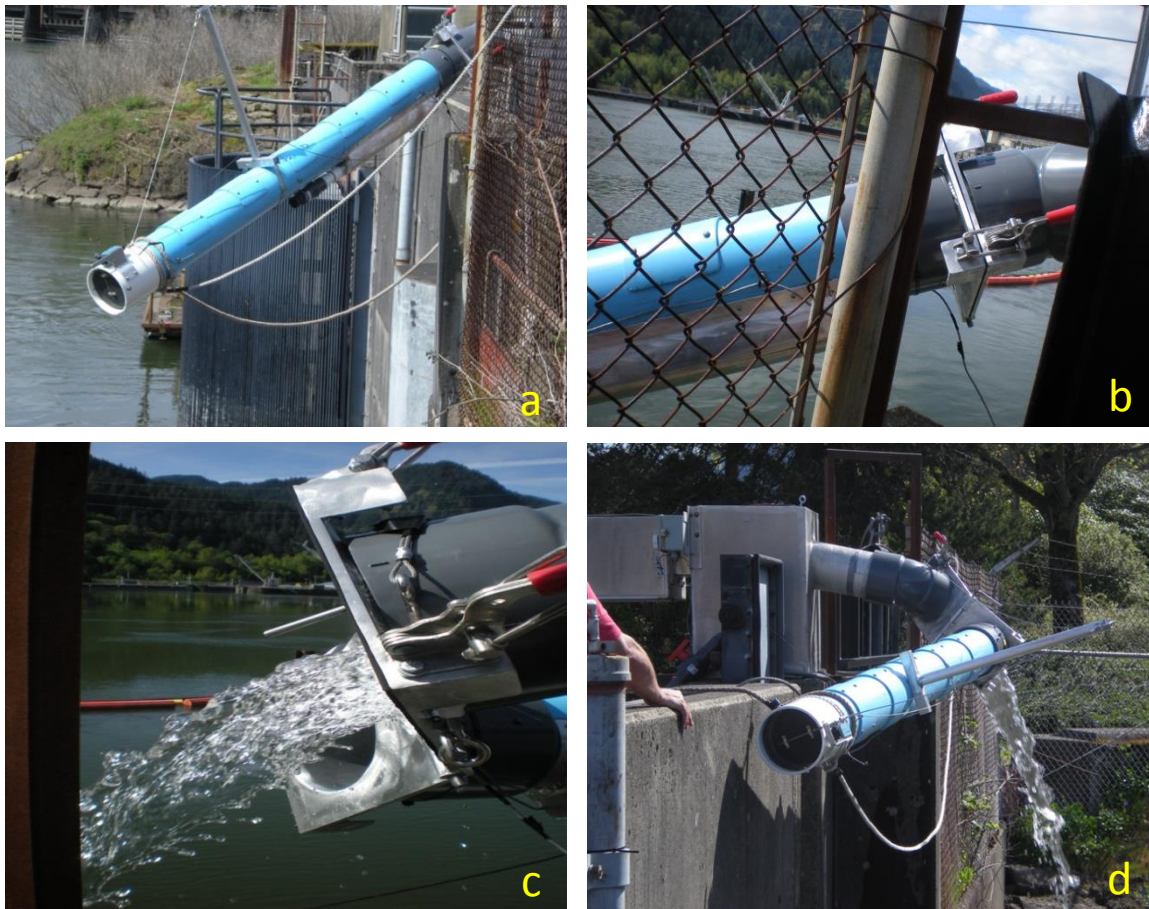
Figure B10. Retractable exit slide of Bradford Island LPS showing slide deployed (a), hinge closed (b), hinge open (c), and slide retracted (d).
