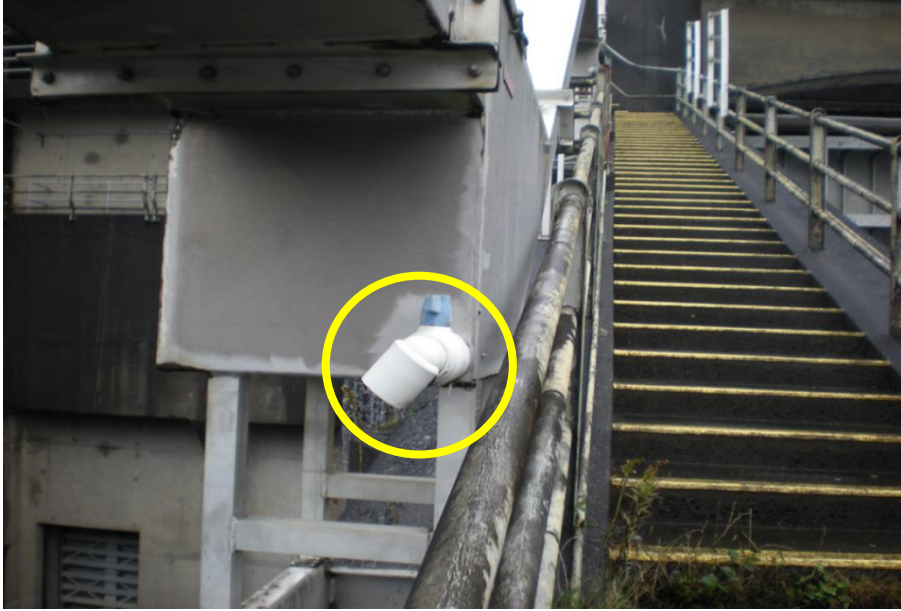
Figure B6. Example of a discharge valve at a rest box.
