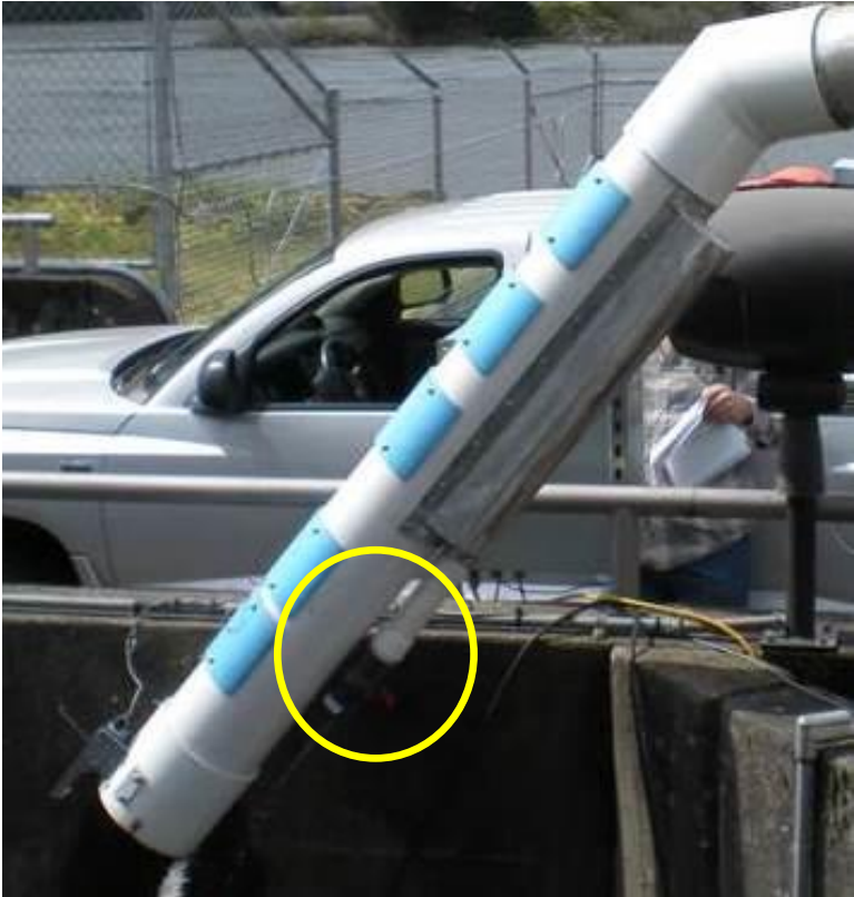
Figure A5. Discharge valve at exit slide of Washington Shore AWS LPS.
